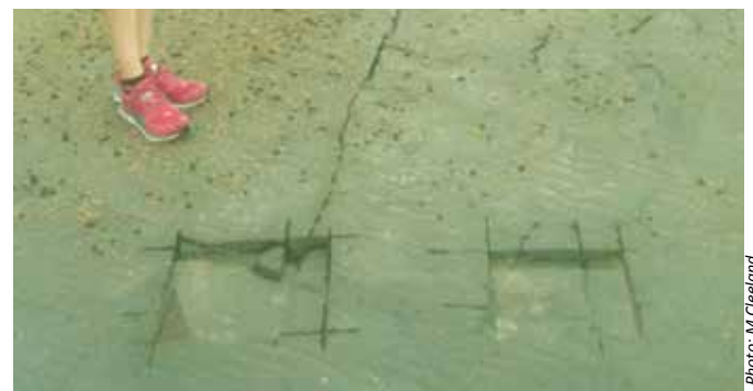
Saw-cuts show the position of the footprints at Browns Creek
