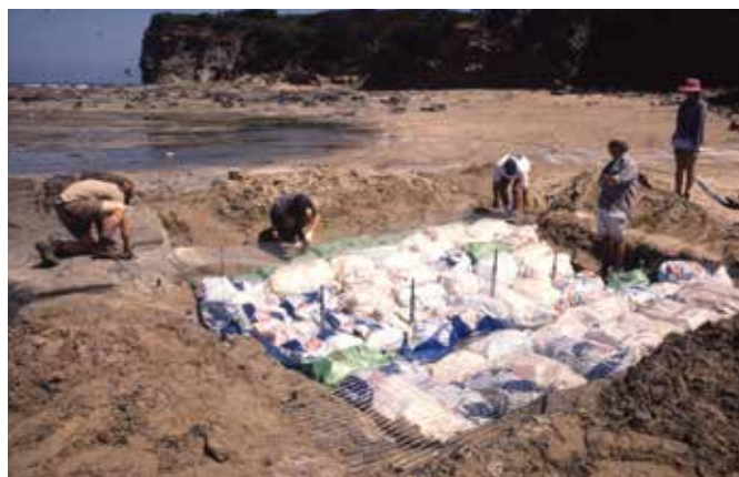
The System is installed in 1998
