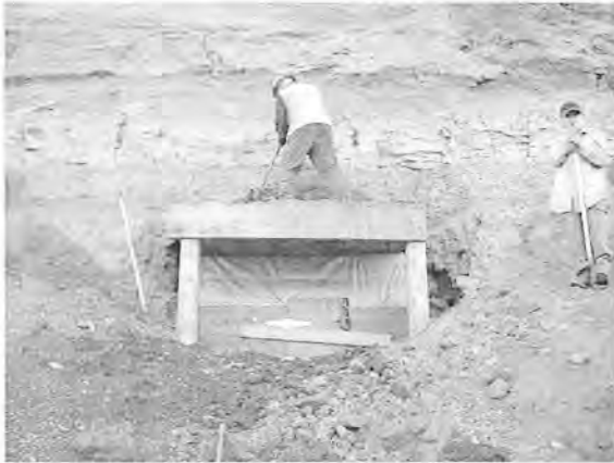
Clearing debris from the portico
