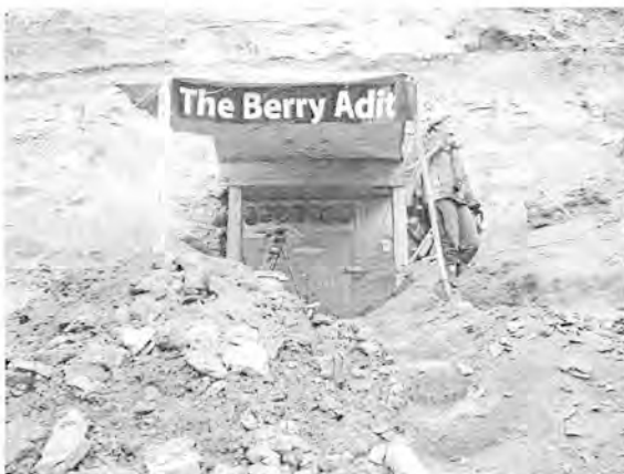
The Berry adit ready for floor excavation
