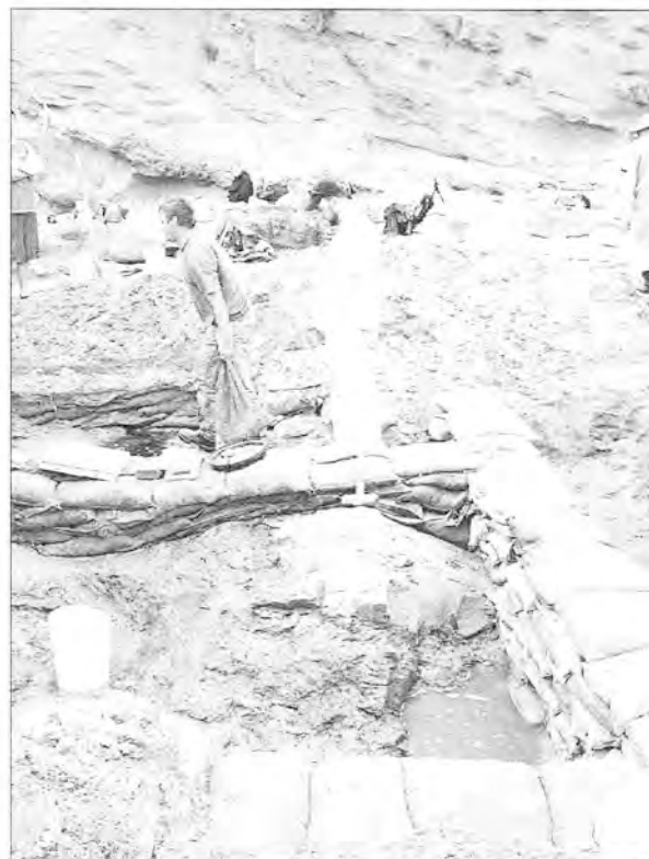
John Swinkels and Troy Radford helping to rebuild the sandbag walls after the System was dismantled.
