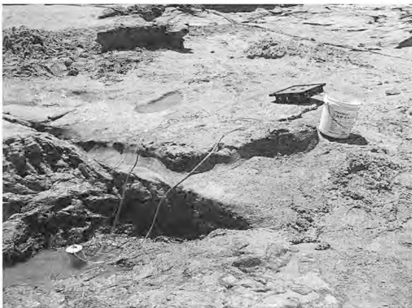
The solar pump in operation
